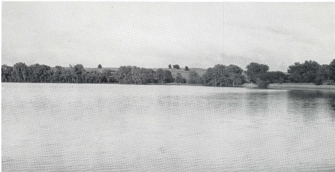
A view of Ottawa County State Lake with the dam and spillway on the right.
